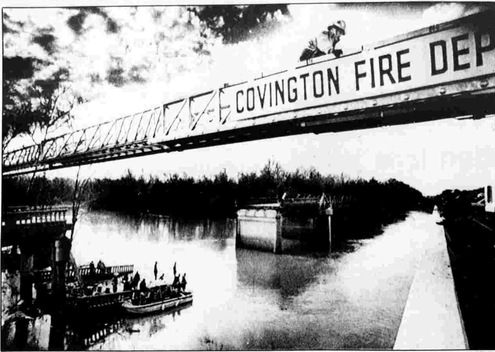
WHERE 7 DIED — A firefighter carefully makes his way back across an aerial ladder from part of the still-standing U.S. 51 highway bridge across the Hatchie River in Covington, Tenn., Sunday. At least seven people were killed when the 60-foot section of the half-century-old bridge collapsed late Sunday. Workers near the water are searching for bodies.
